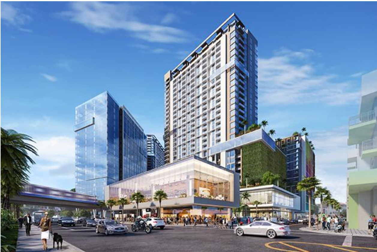
The Link at Douglas is an example of transit-oriented development coming to the Miami area. The mixed-use project is being developed jointly by 13th Floor Investments and The Adler Group at Miami-Dade County's Douglas Road Metrorail station in Coral Gables.
