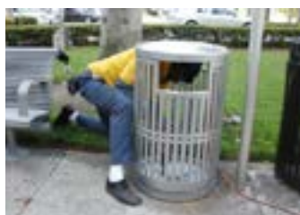
DET - Trash Receptacle Installation in Brickell
