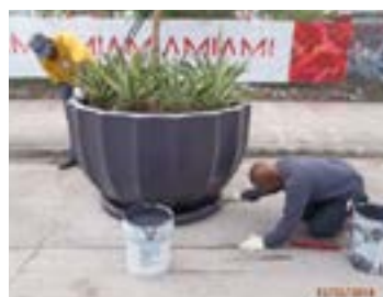
DET - Planter Repair & Maintenance
