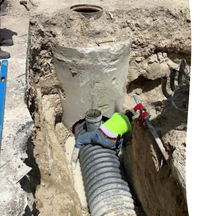
• Sealing 24" HDPE drainage pipe to drainage structure S-38.
