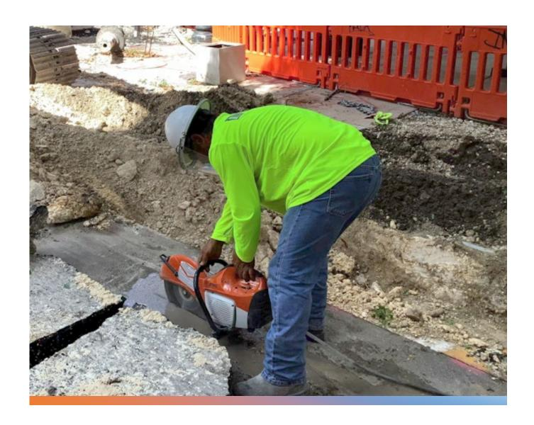
Saw cutting asphalt pavement for removal
