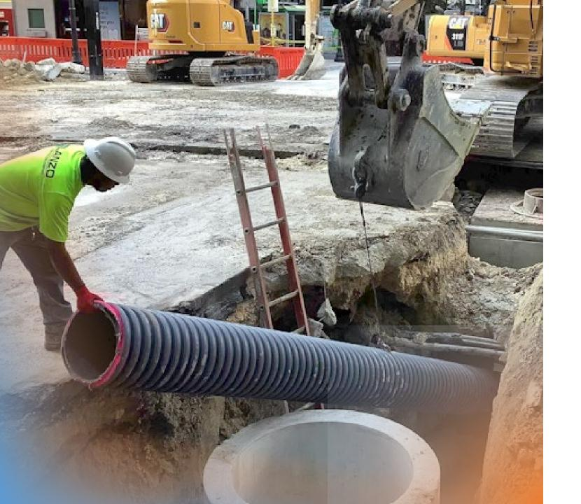
• Installing 15" HDPE drainage pipe between S-34 and S-32
