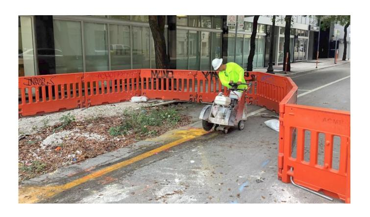
Saw cutting asphalt pavement for excavation
