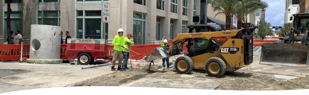
• Back filling trench with lime rock material.
