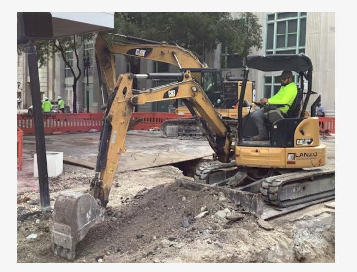
• Excavation of materials for drainage pipe.
