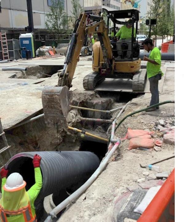
• Installation of 24" HDPE drainage pie
