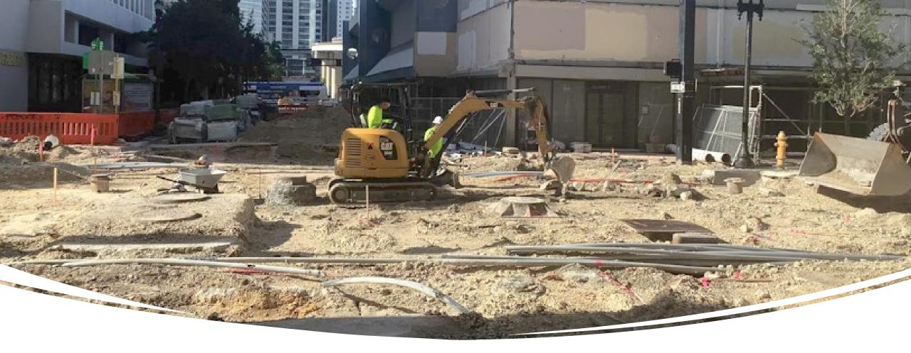
• Removing existing manhole to adjust new manhole to finish grade
