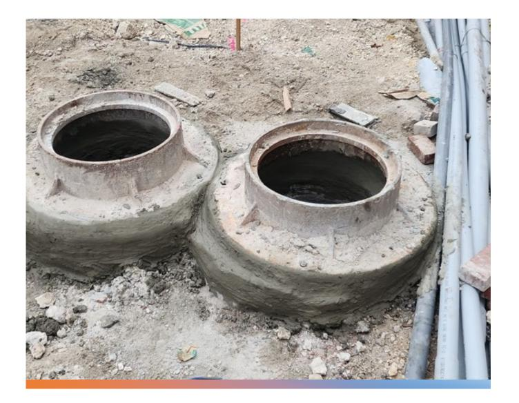
• Installed and sealed manholes for drainage structures.
