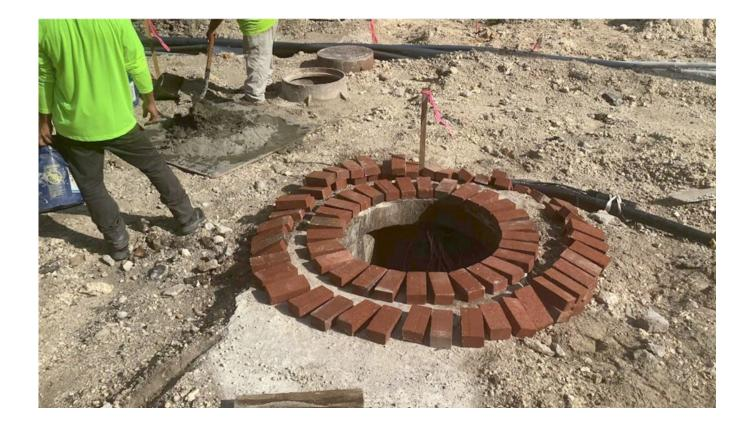
• Installing brick pavers to adjust manhole elevation for drainage structure
