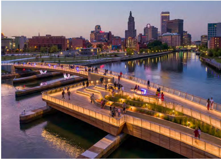
Michael S. Van Leesten Memorial Bridge – Providence, RI
