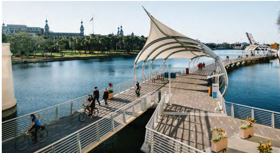
Tampa Riverwalk – Tampa, FL
