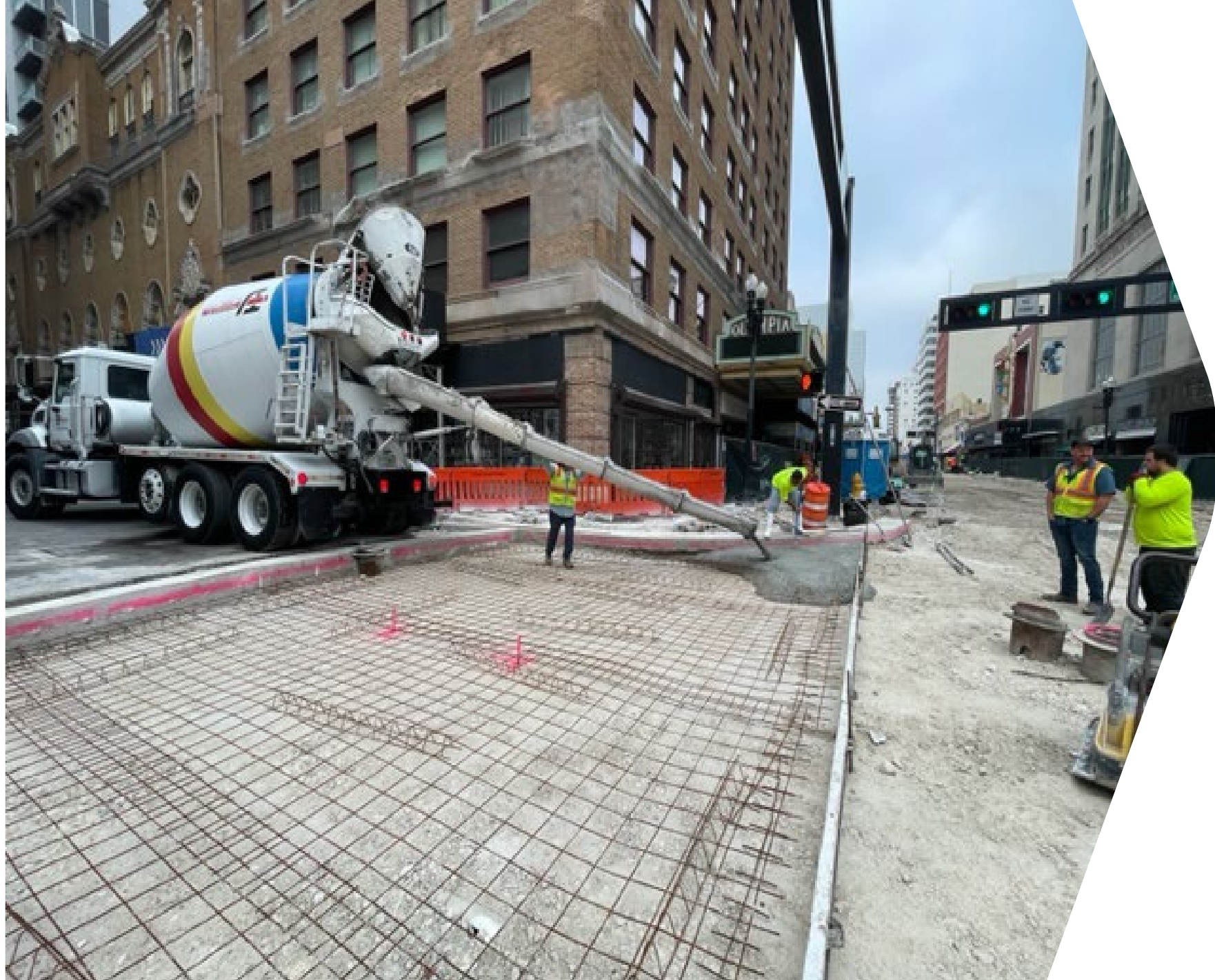
Phase C (E 2 nd Ave to E 1 st Ave) Intersection at E 2 nd Ave Roadway Concrete Slab
