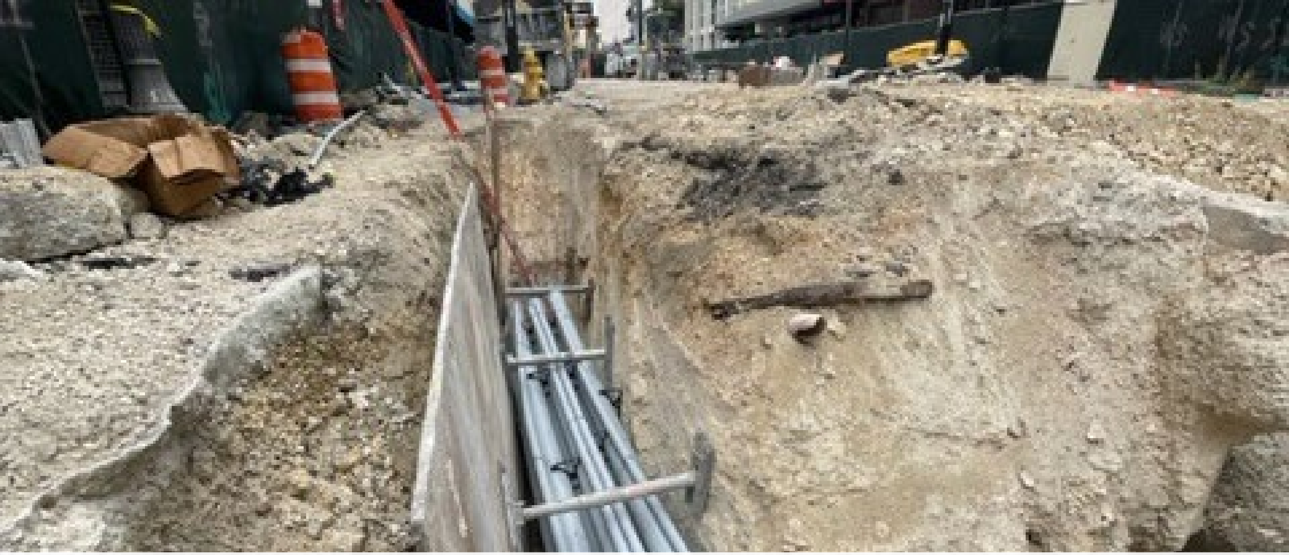
Installation of FPL duct bank
