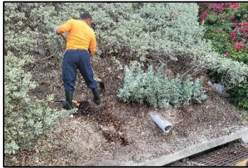
NEAT Gateway Maintenance
