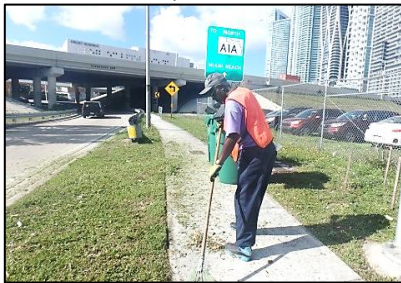
DET/CRA ROW Maintenance
